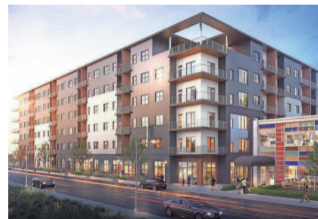
TWG Development will build more than 150 apartments along the Red Line at 1827 N. Meridian St. COURTESY OF TWG DEVELOPMENT
