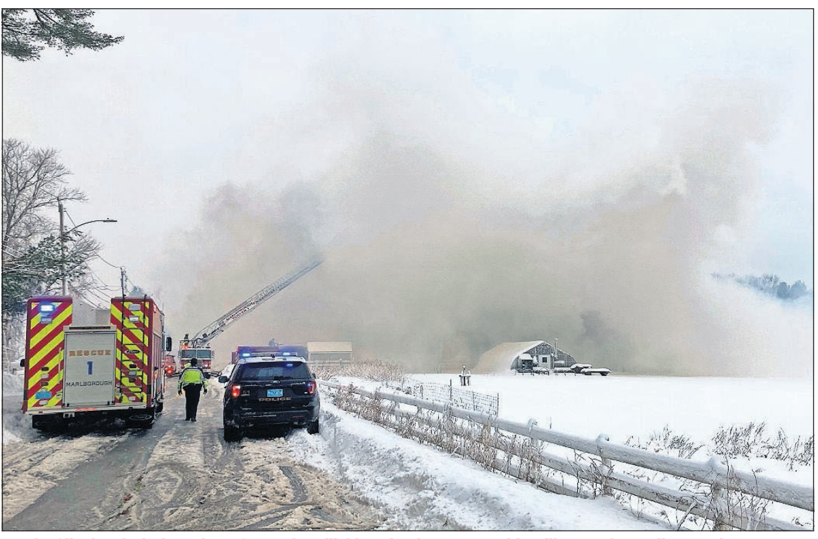
Smoke fills the air during a barn fire at the Hillside School Farm on Robin Hill Street in Marlboro, Feb. 2, 2021. Much of the barn has already collapsed. [DAILY NEWS AND WICKED LOCAL STAFF FILE PHOTOS/ART ILLMAN]
