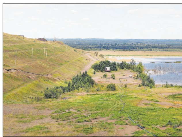
Steve Kuchera / 2017 file / Duluth News Tribune Plans for PolyMet include building dams to increase the storage capacity of tailings basins. One would be built in the distance to raise the basin on the right to the level of the area on the left.
